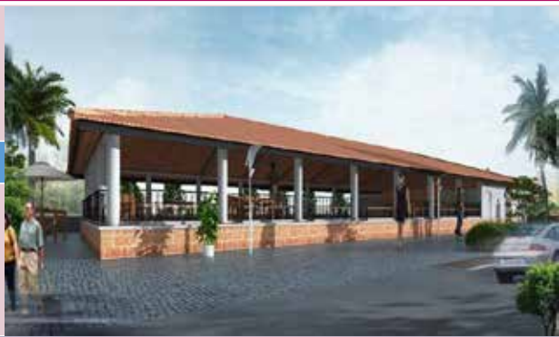
VIEW ON COMPLETION
