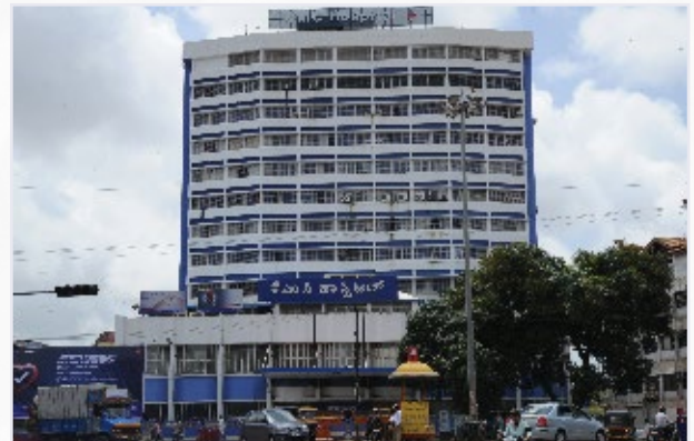
KMC Hospital Ambedkar Circle, Mangalore
