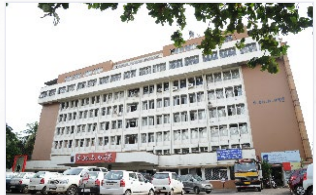
KMC Hospital, Attavar, Mangalore
