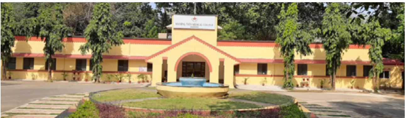
New Manipal TATA Medical College, Jamshedpur (Phase -1 work)
