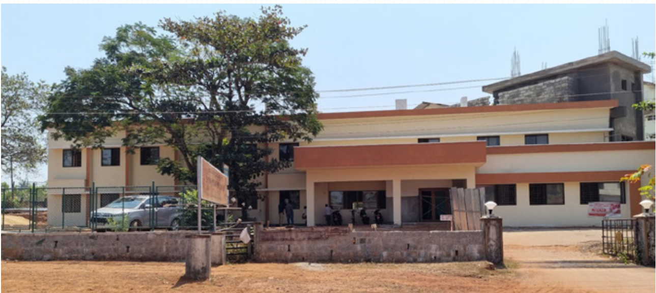
Expansion of TMA Pai Rotary Hospital at Karkala
